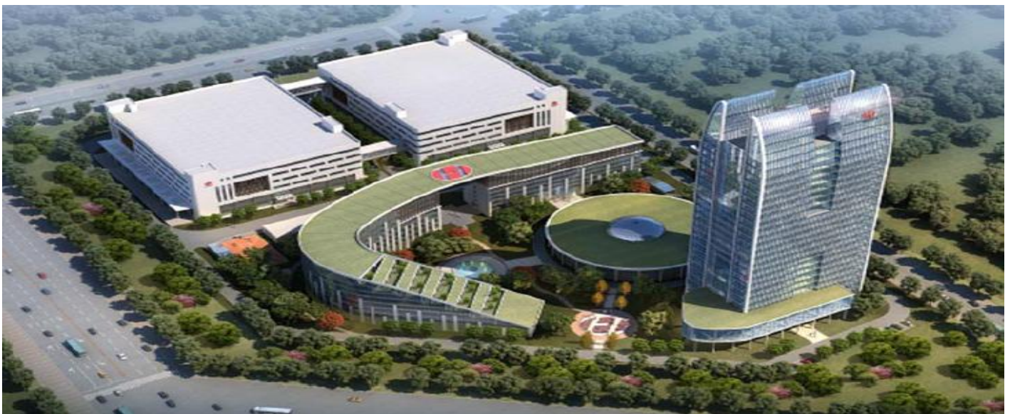
New HQ in Wuhan, under building
